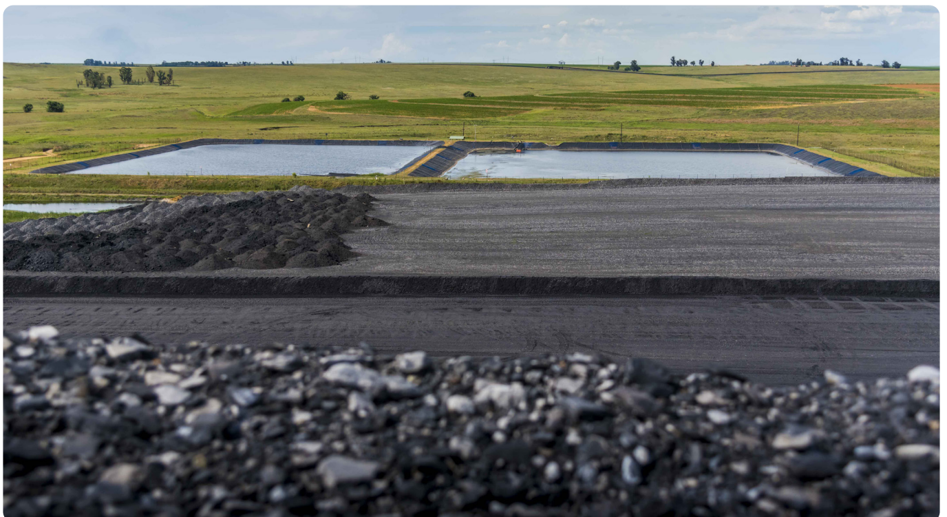
Pollution control dams at our ECC operation which Exxaro exited in September 2021
