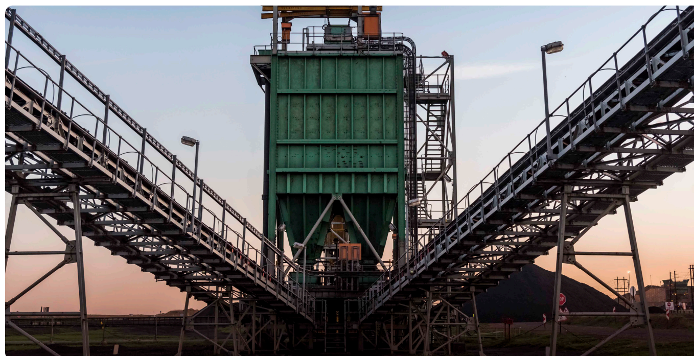
Silo at ECC
