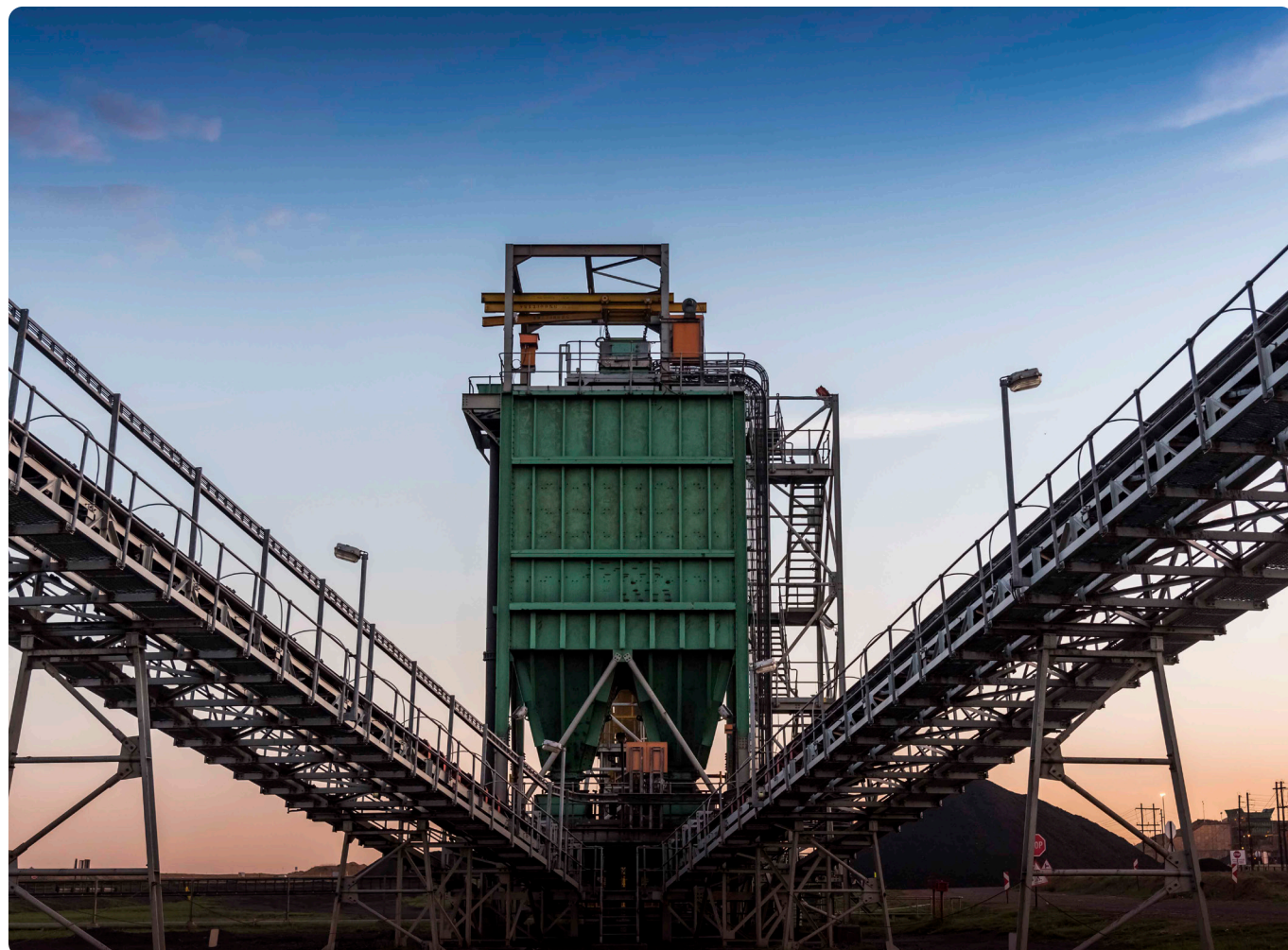
Silo at ECC
