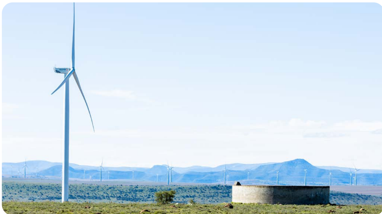
Amakhala Emoyeni windfarm between Bedford and Cookhouse in the Eastern Cape
