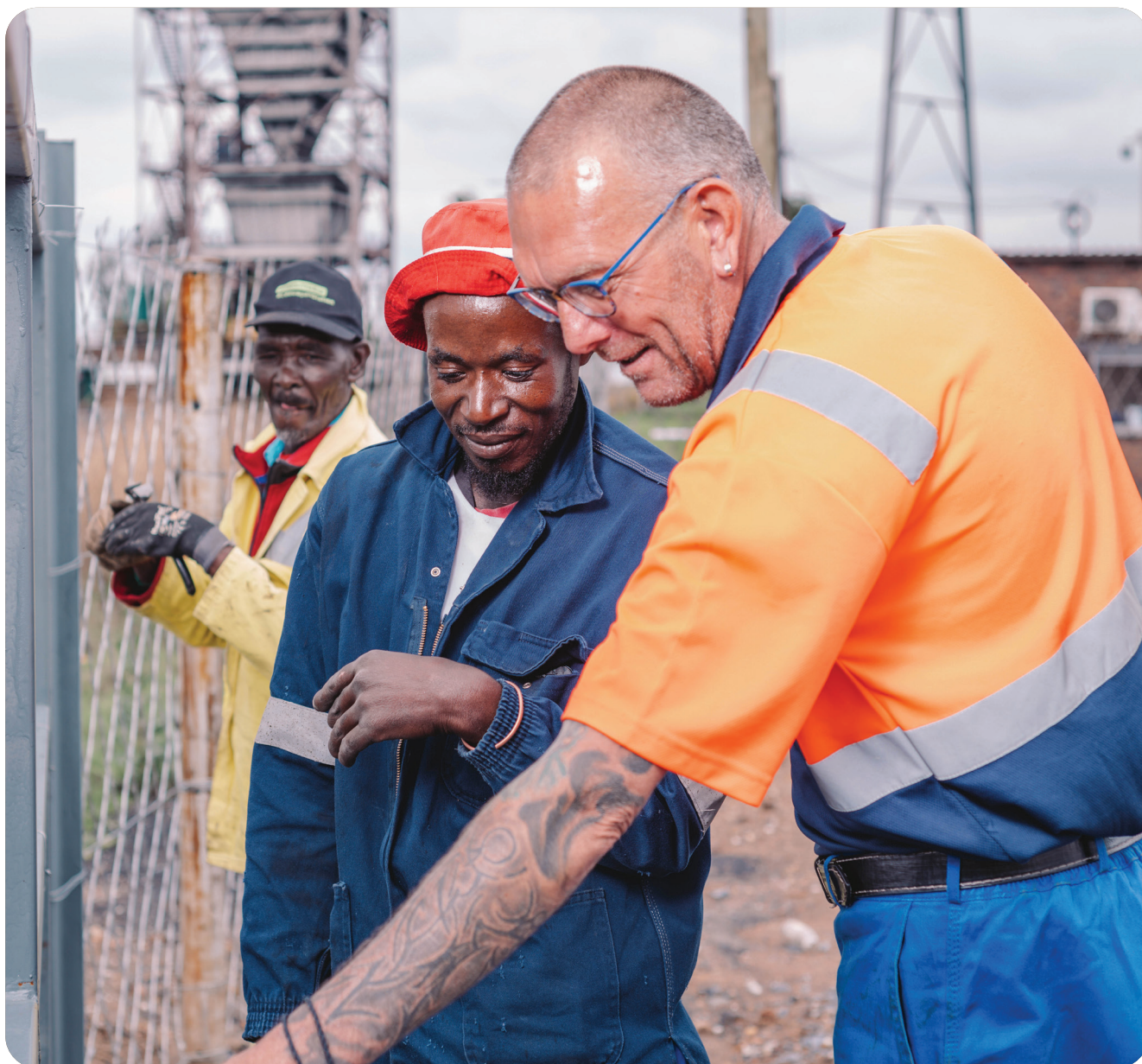
Exxaro maintenance team at work
