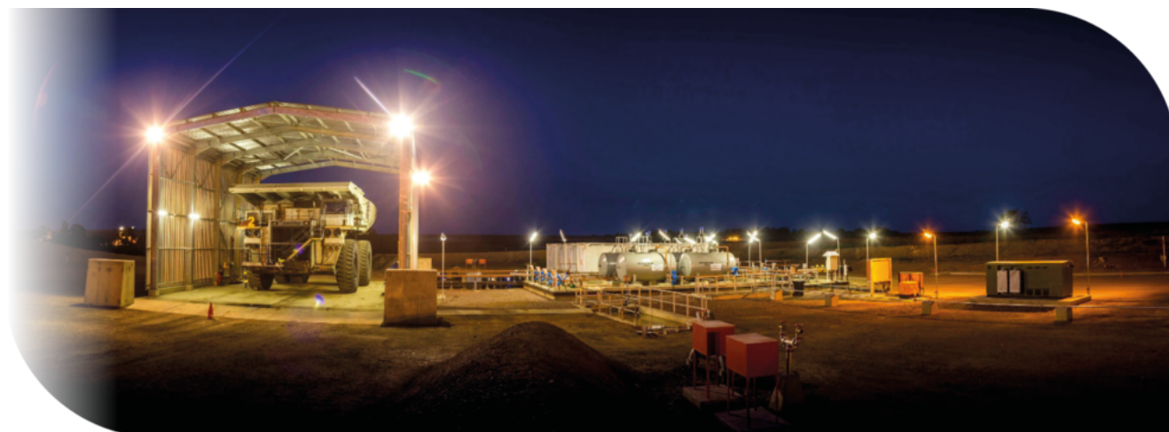
Service bay for production trucks
