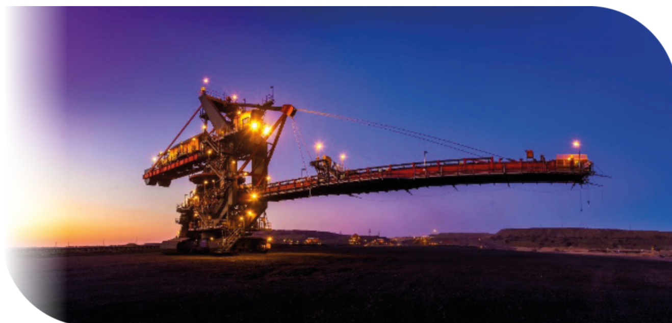
Stacker for discard backfill at Grootegeluk
